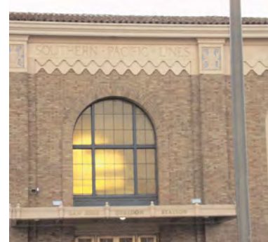
Brickwork on the 1920s Cahill/Diridon train depot.
