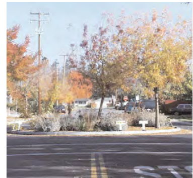
Traffic circles can serve to calm traffic and feature attractive landscaping.
