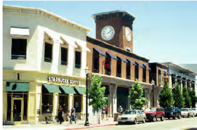
A consistent frontage of neighborhood-oriented commercial businesses is recommended for West San Carlos Street.
