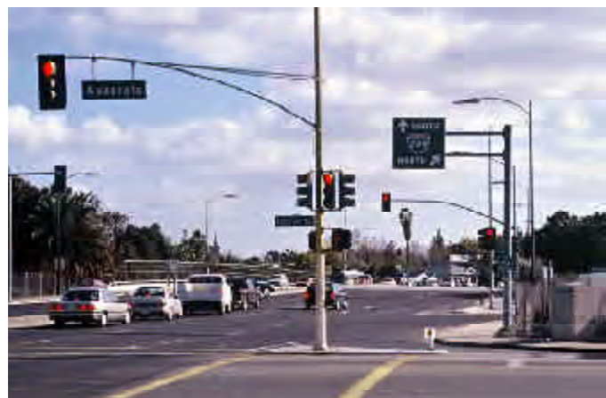
Safety and visibility of pedestrian crossings at freeway ramps needs to be enhanced.
