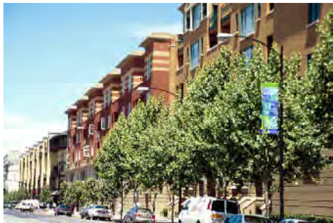
Infill housing averaging 4-5 stories in height should be considered along West San Carlos Street.
